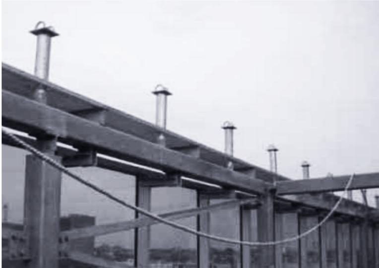
We offer a variety of single-point fall protection anchors, from rigid to tip-over style to portable solutions. System types also include D-ring single point anchors, fixed truss anchor kits, and portable truss anchor kits.
