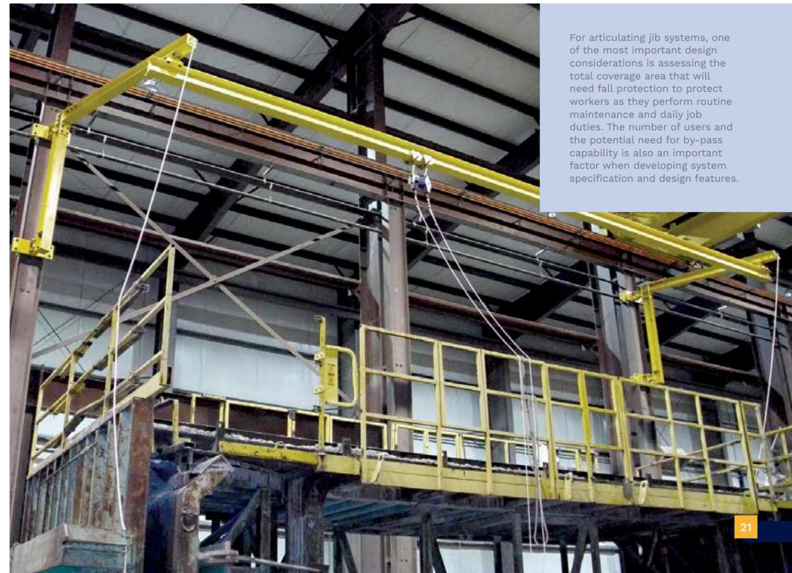
For articulating jib systems, one of the most important design considerations is assessing the total coverage area that will need fall protection to protect workers as they perform routine maintenance and daily job duties. The number of users and the potential need for by-pass capability is also an important factor when developing system specification and design features.
