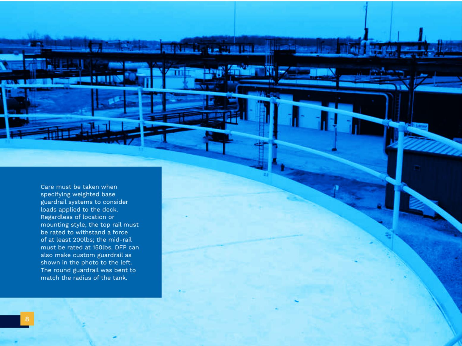
Care must be taken when specifying weighted base guardrail systems to consider loads applied to the deck. Regardless of location or mounting style, the top rail must be rated to withstand a force of at least 200lbs; the mid-rail must be rated at 150lbs. DFP can also make custom guardrail as shown in the photo to the left. The round guardrail was bent to match the radius of the tank.
