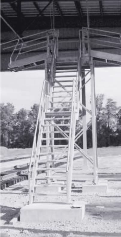
Access platforms, stairs, and gangways are simple, easy-to-use passive fall restraint systems designed to prevent slips and accidents before they happen. Access platform designs can range from single station installations to complex, multi-unit systems. (For loading and unloading applications, the access platform's height must allow sufficient clearance for railcars, tankers, and trucks commonly serviced.)
