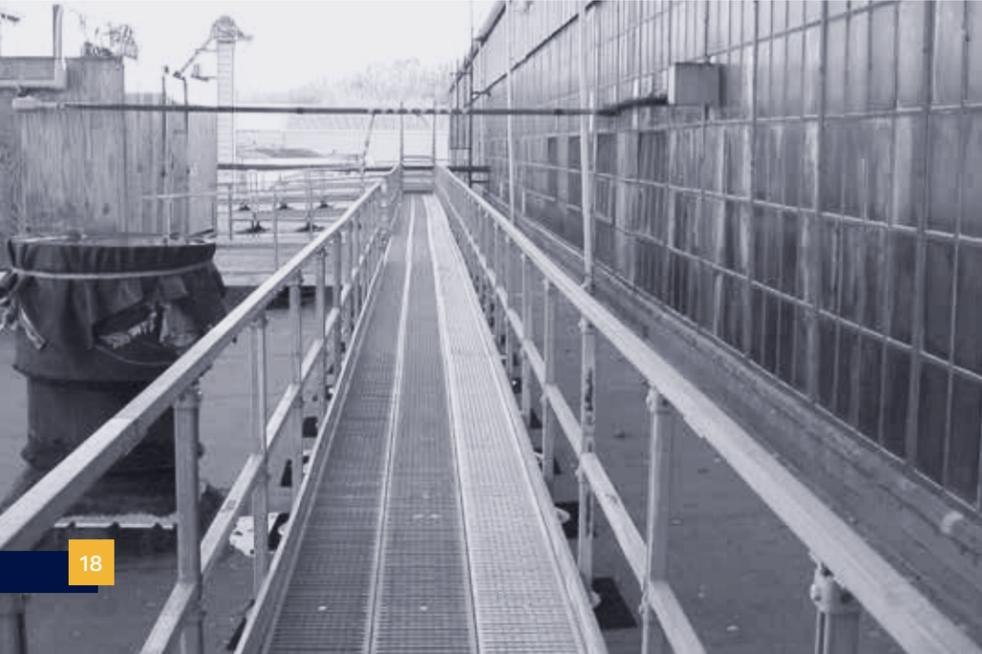
Resisting outdoor conditions in galvanized steel or aluminum finish and attaching to a variety of roof types, Rooftop Walkways and Crossovers are available factory-assembled or assembled on-site and these OSHA-compliant systems are ideal for most rooftop maintenance activities or traffic.
