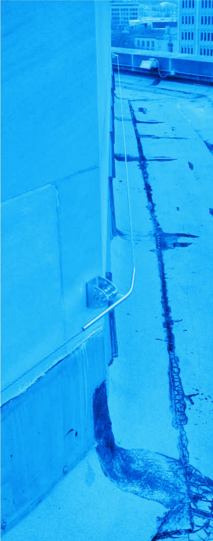
The slope and the construction of your roof are the two factors when determining your rooftop lifeline. No matter the style, all DFP lifelines are a continuous pass-through system that allow workers to travel the entire system length without disconnecting.
